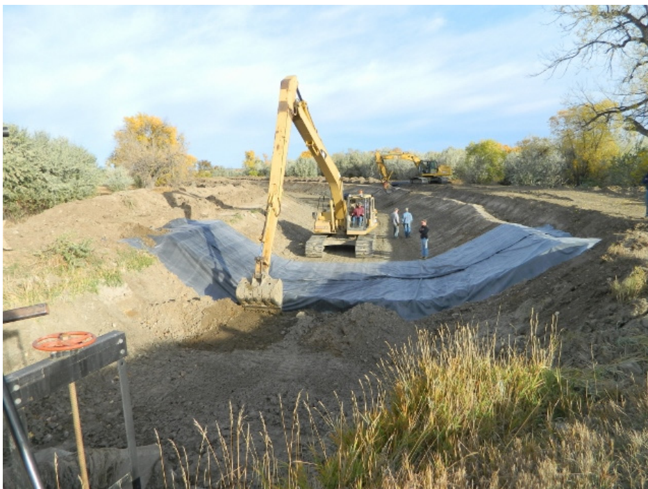
Figure 3-4. Lining the South Canal.
